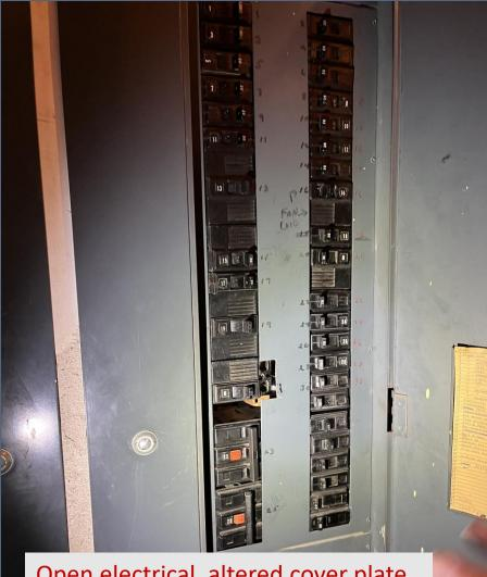
Open electrical, altered cover plate, multiple tripped breakers
